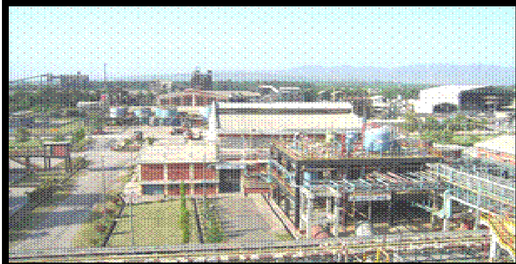
Aerial View of Plant
