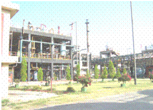
Caustic Soda Concentration Unit & Boiler
