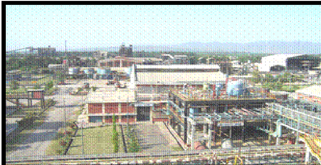
Aerial View of Plant
